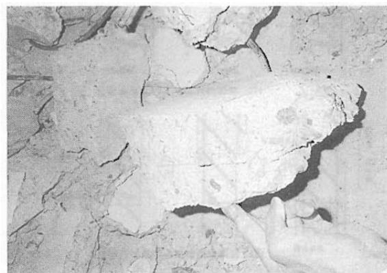
Photo 11 Part a Reinforced Concrete Wall, Demolished in Flakes of Size Easy to Remove.
