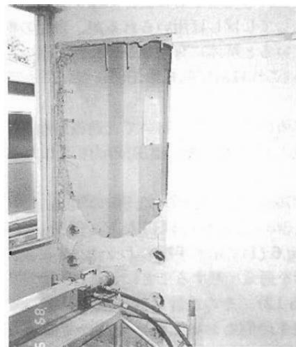
Photo 10 Removal of a Part of a Wall to Secure an Opening Where a Door Will Be Installed. After Electric Heating of Reinforcing Bars, Concrete Is Removed by Secondary Break-up Work Using a Hydraulic Jack.
