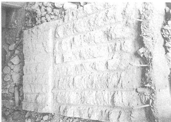
Photo 3 Concrete Surface of Remaining Wall after Removal of Covering Concrete and Heated Bars. Bars are Completely Removed as Well.
